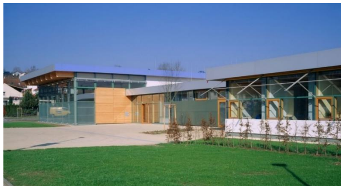
Figura 7 Vista Exterior-Pistorius School for Disable Children
